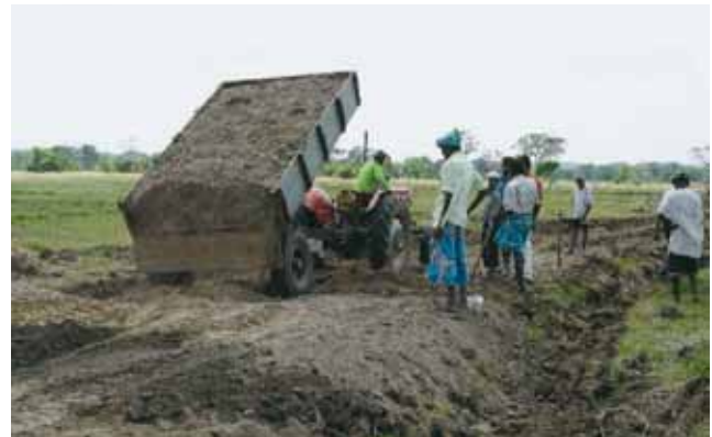
Rehabilitation of rural infrastructures by the community people (Agriculture road)
