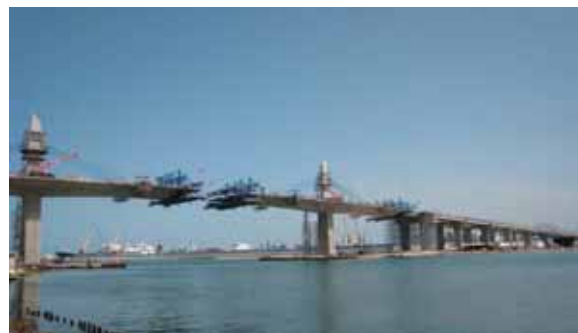
Main and South Approach Bridges under construction
