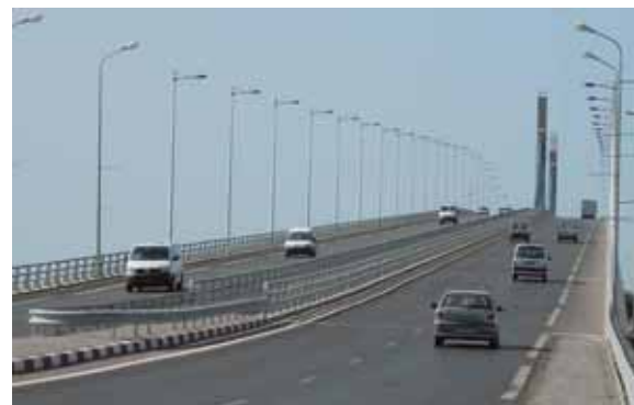
South Approach Bridge
