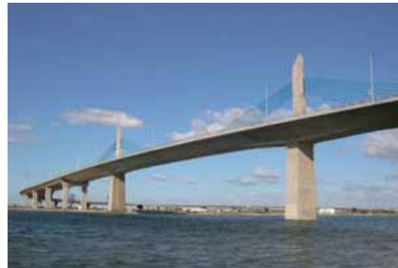
Main Bridge, North Interchange and Ramp Ways
