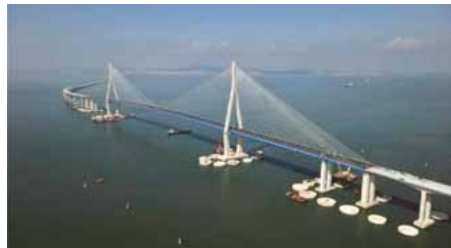
Completed Incheon Bridge
