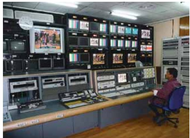
Master Control Room
