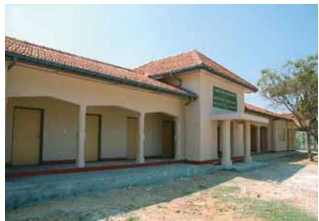
Strengthening of Government Services (Reconstruction of Agrarian Service Center)
